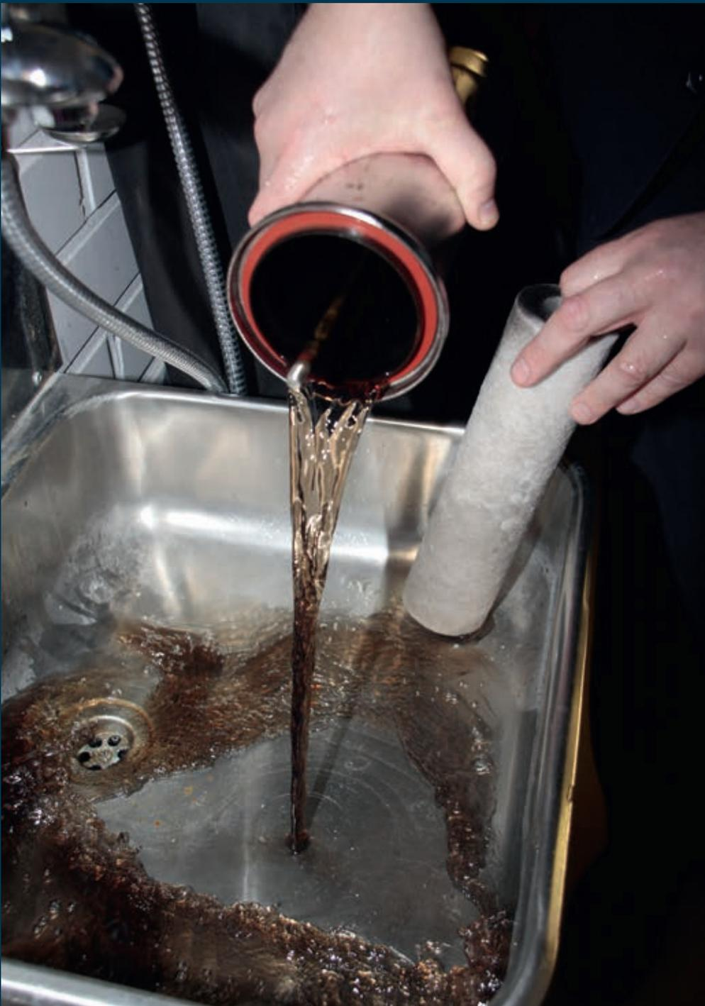
The filter is changed when necessary, initially a few times a year.
