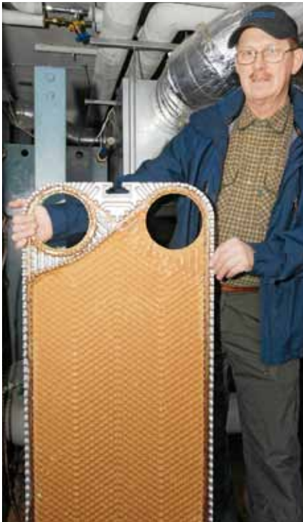
– This is how the plates of the heat exchanger used to look like. They had to be cleaned regularly – in total 3-4 times between 1986-2008, describes Stig Kyldén, vice chair of the housing association in Skövde.
